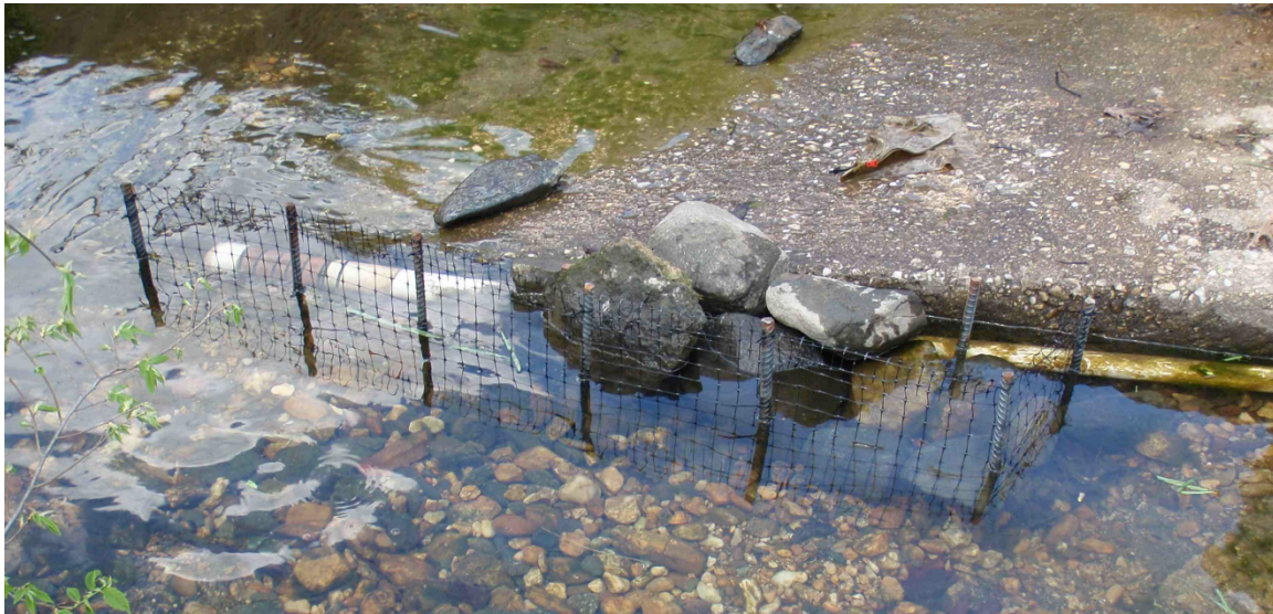
Figure 20. Example protective cage made of deer fencing and rebar.
